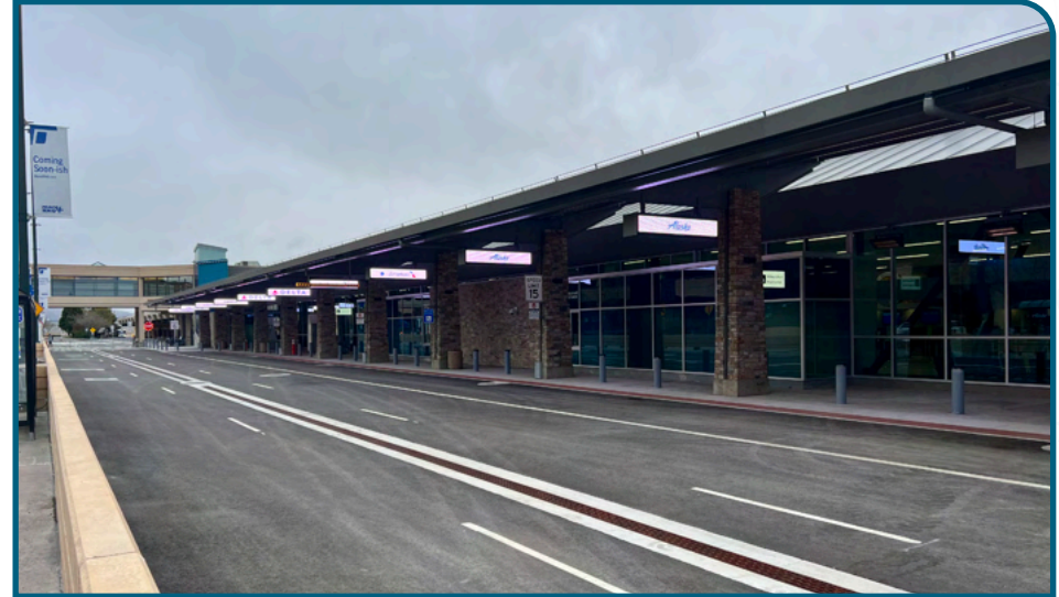
Completed Terminal Loop Road - Departures Side
