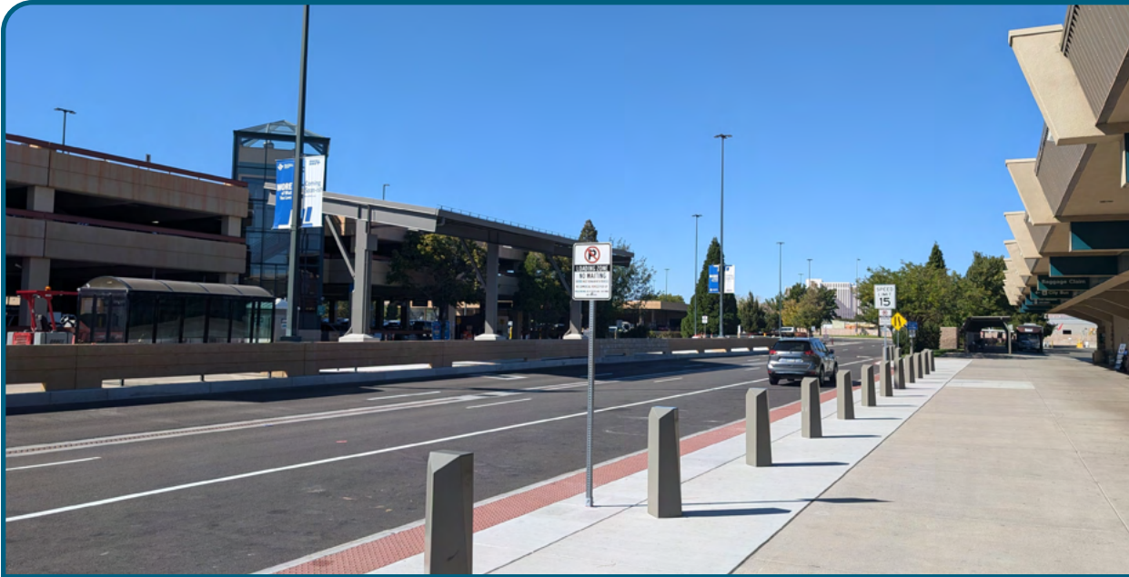
Bollards Installed at RNO
