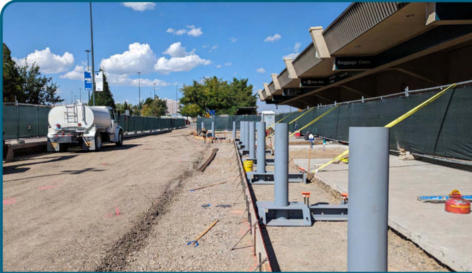
Terminal Loop Road During Construction - Departures Side
